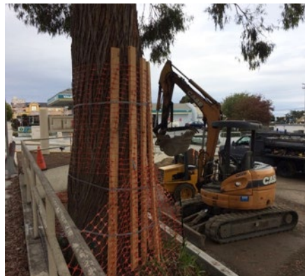
Figure 3. Grade changes from construction can result in major root system injury.
