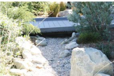
Figure 5. This dry streambed channels runoff from roof downspouts to vegetated areas a safe distance from the building.
