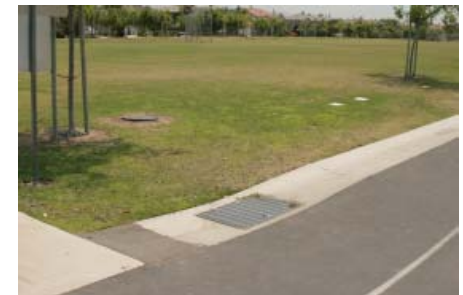
Figure 4. This exposed landscape drain, which is located adjacent to a large sports field, can easily carry pesticides to storm drains and local bodies of water.
