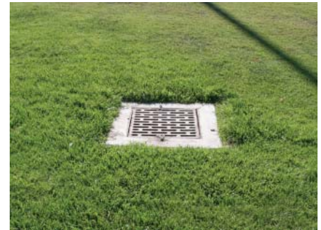
Figure 2. Landscape drain located in the center of a large park turfgrass area.
