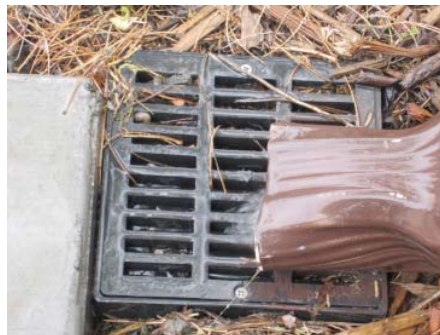
Figure 3. Downspout draining directly into a landscape drain.
