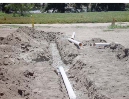
Figure 6. Installing perforated drainage pipe helps reduce waterlogged soil.
