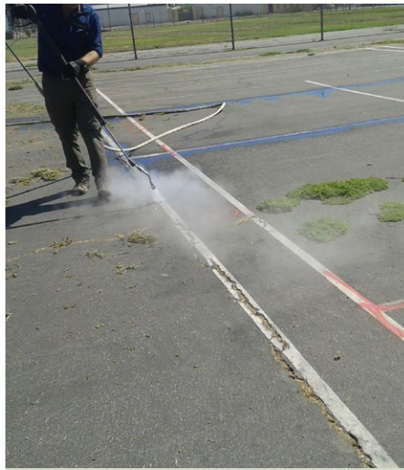
Figure 6. Pressurized steam being used to kill weeds growing in cracks in a school playground.
