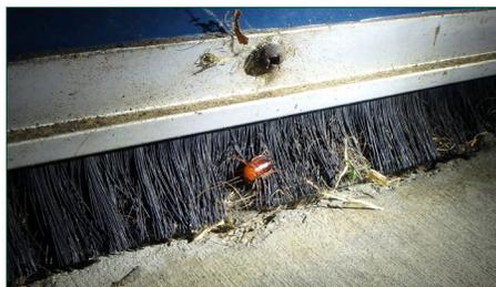
**Figure 13. Install door sweeps on exterior doors to prevent outdoor cockroaches from entering structures.**
