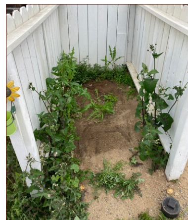
Figure 2. Weeds and other flammable materials next to fences can create a fire path to the siding or the eaves of a house.
